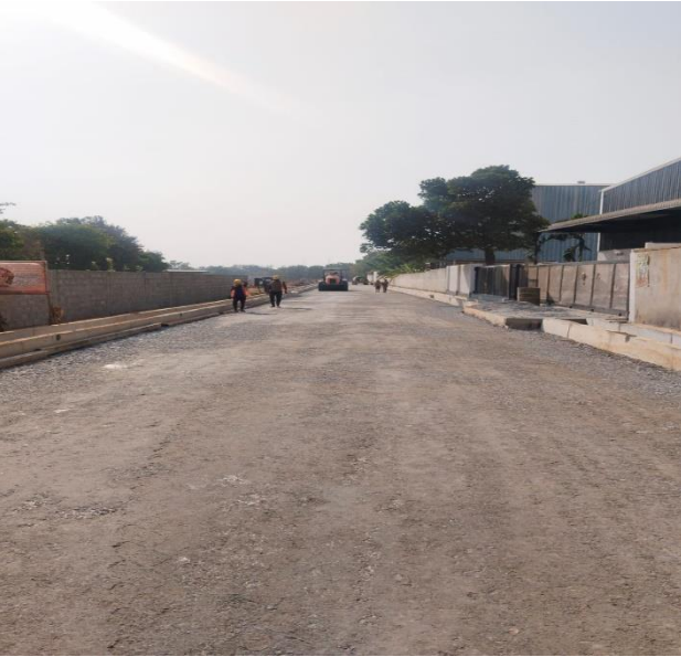
Phase-2 Nelamangala rural road infrastructure upgradation
