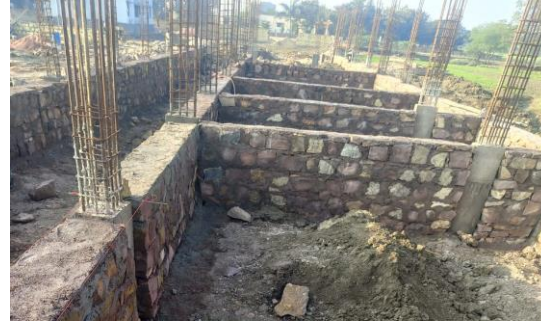
Construction Support – Government School
