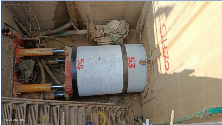
Ahmedabad microtunneling project in Gujarat
