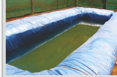
RAIN WATER HARVESTING
