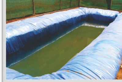
RAIN WATER HARVESTING
