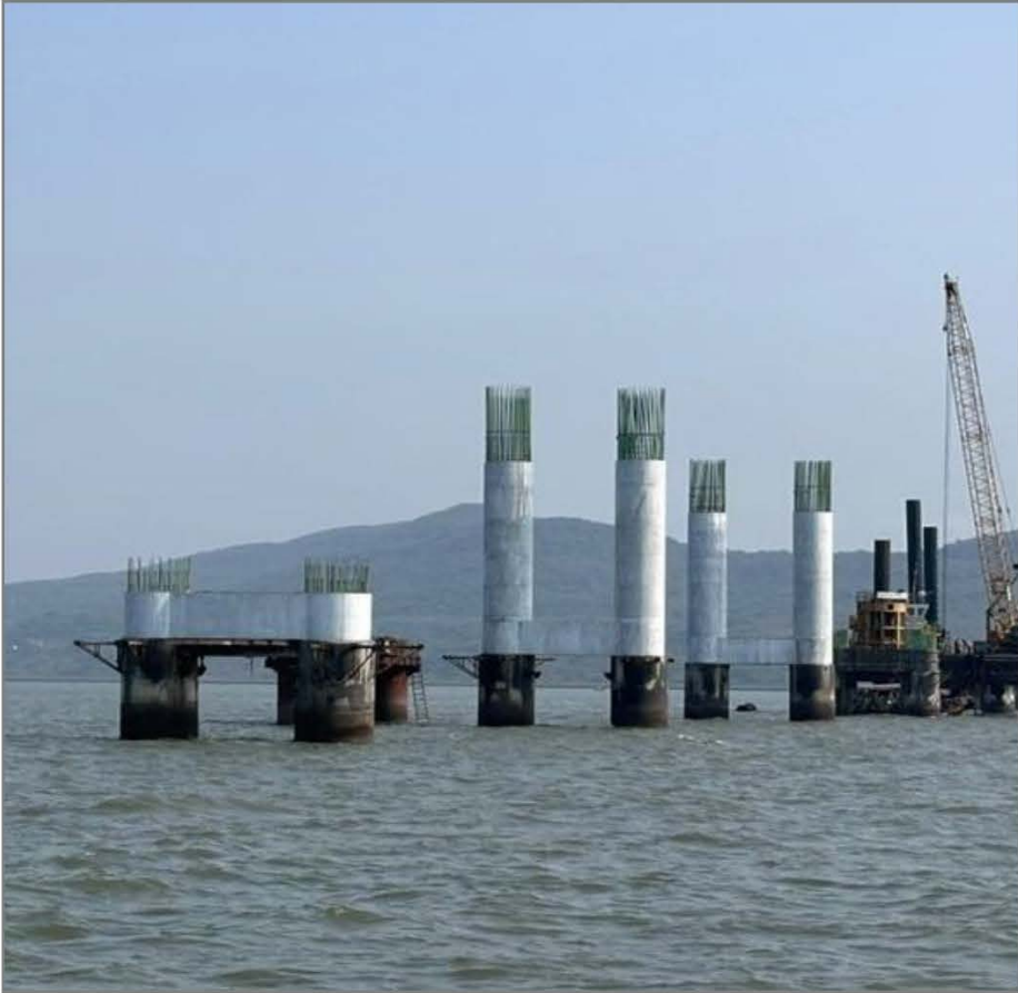
Pile, Crossbeam and Pier between P30 to P33
