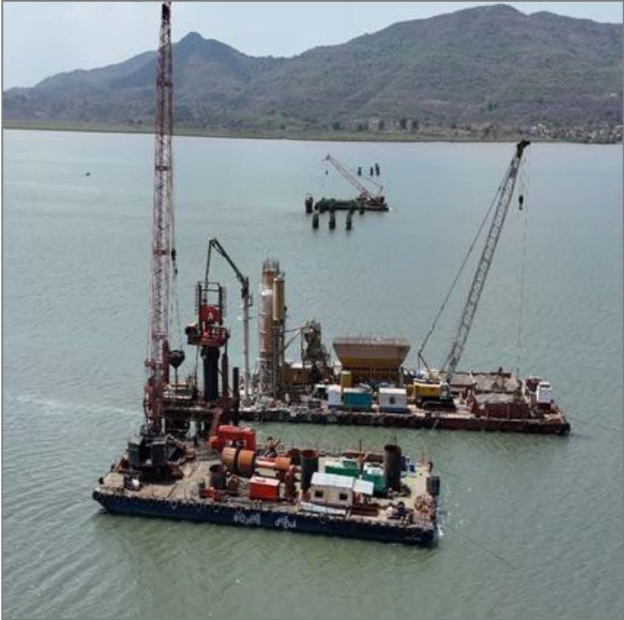
Floating Batching Plant
