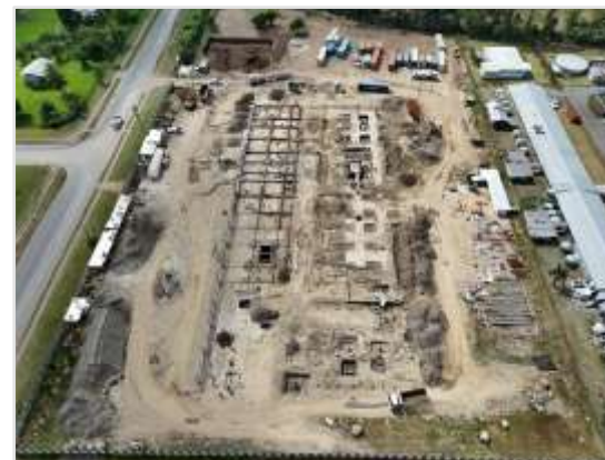
Hospital Construction Progress
