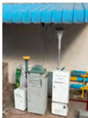
AAQ Station installed in Vadakuvellore, Neyveli
