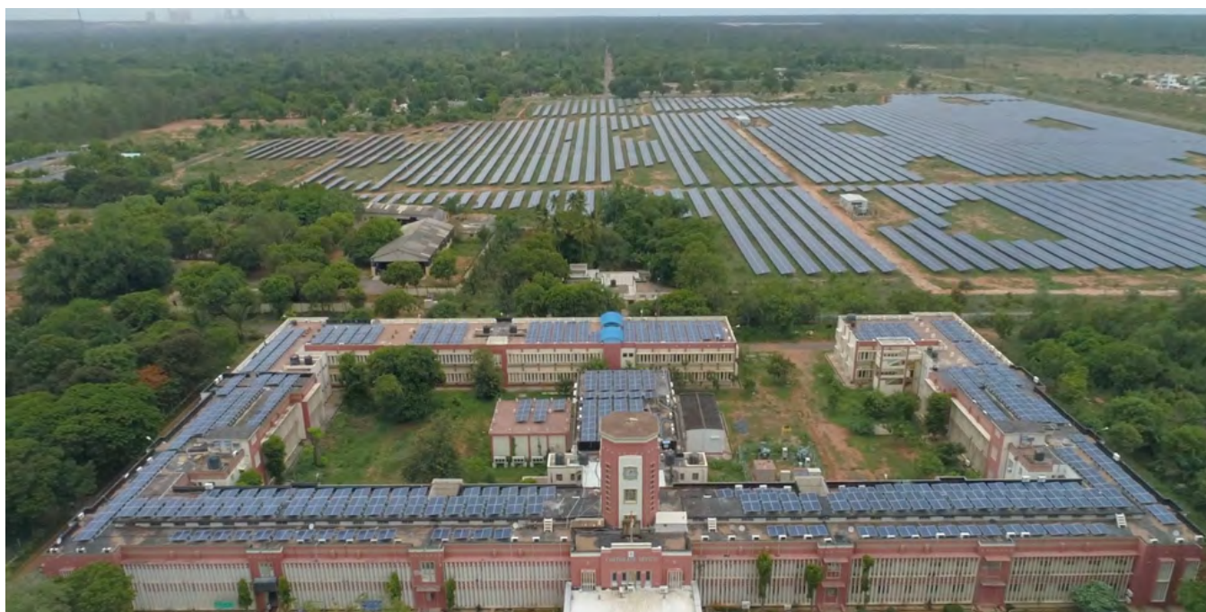
Rooftop Solar Plant at Corporate Office, Neyveli
