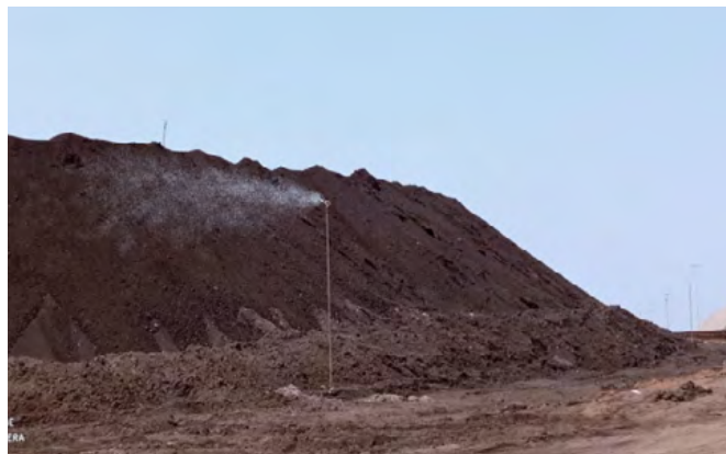
Spray Guns in Bunker Area
