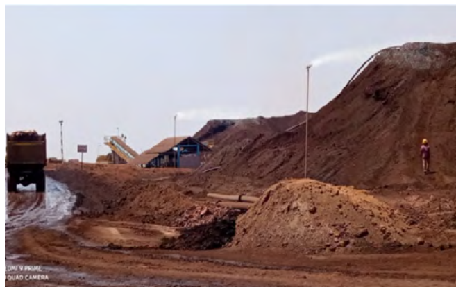
Vehicular Water Spraying
