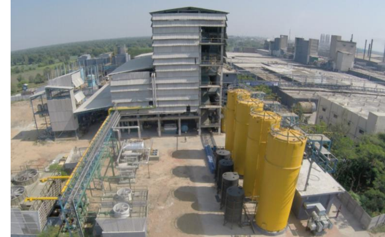
Multiple Effect Evaporator Plant (MEEP)
