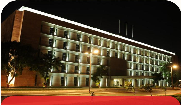
Government Office Building
