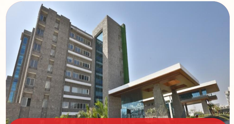
R&D Centre at Vadodara
