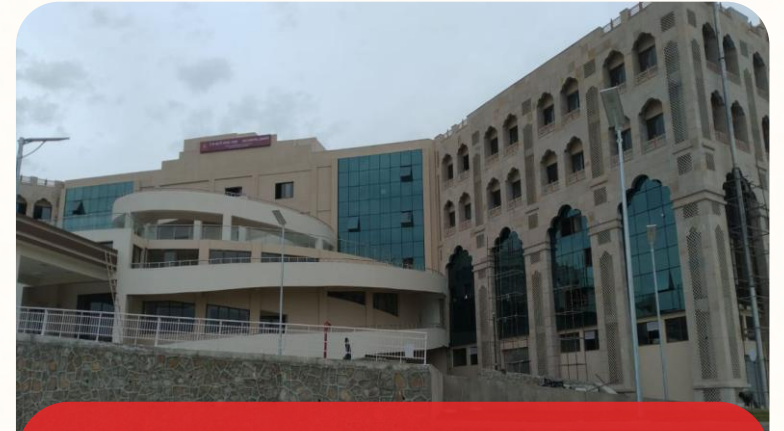
Hospital Project In Udaipur Rajasthan
