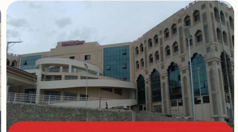
Hospital Project In Udaipur Rajasthan
