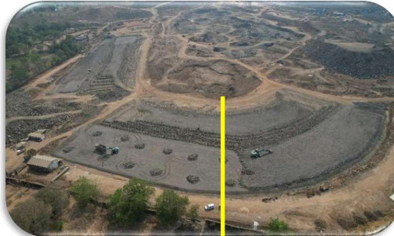
Geomembrane Faced Rockfill Dam
