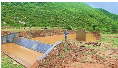
Water Conservation Project
