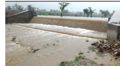
Water Conservation Project
