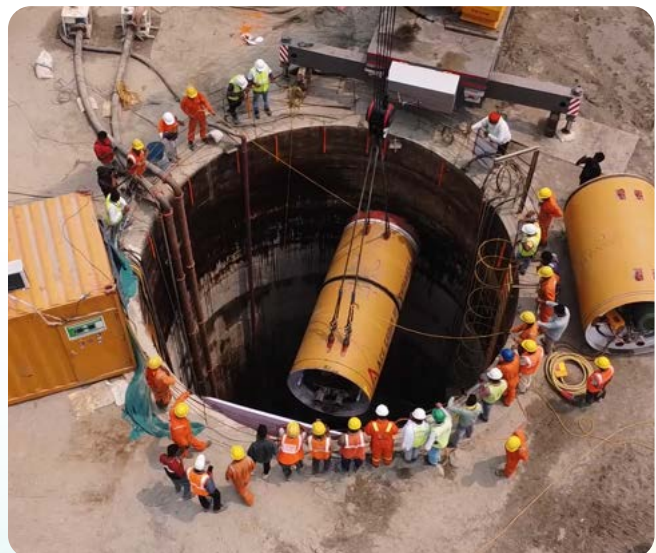
• Pipeline realignment using micro-tunneling technology at Beki river, Barpeta, Assam
