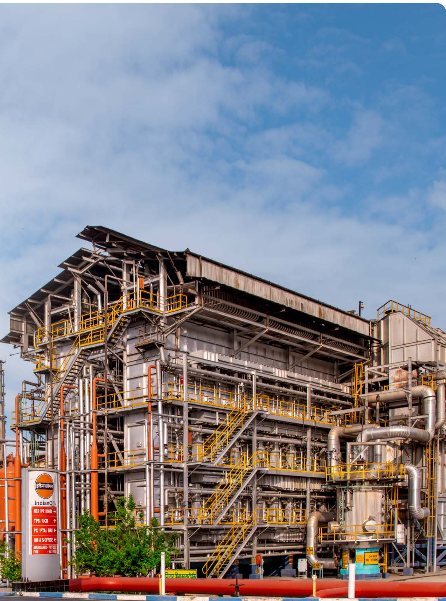
View of Panipat Refinery and Petrochemicals Complex
