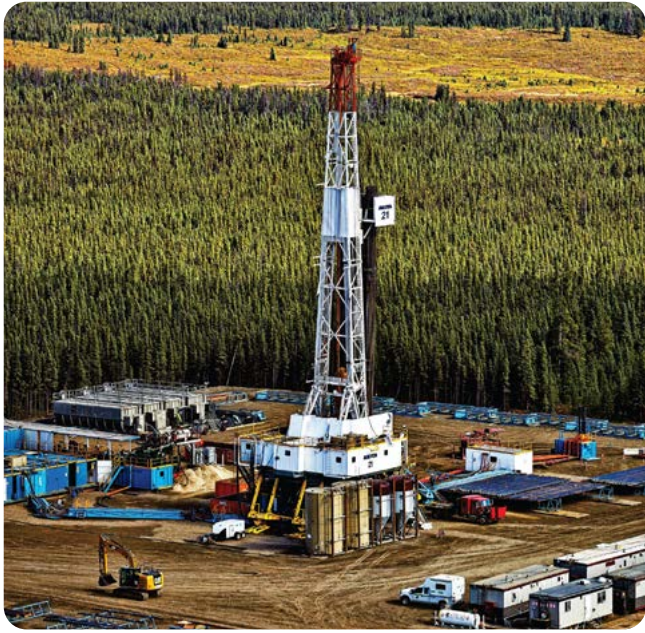
• Rig drilling operations at PNW Akita 21-042, Canada
