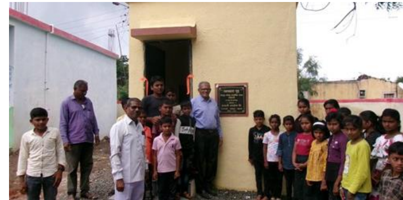
Constructed Toilet Block at Z. P. Primary Center School, Londhewadi, Madha, Solapur dt.10.09.2024
