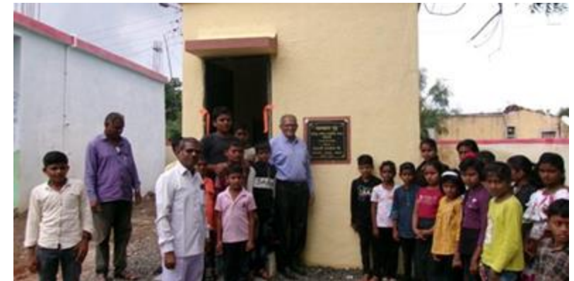
Constructed Toilet Block at Z. P. Primary Center School, Londhewadi, Madha, Solapur dt.10.09.2024
