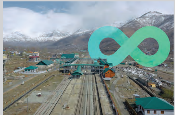
Siemens Limited completed India's first Rigid Overhead Catenary System on the challenging 42-km Kashmir railway route through Pir Panjal range in a record 16 months.
