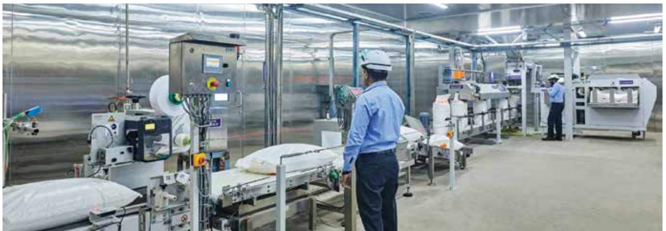
State-of-the-art TAN bagging plant at K-8, Talaja ensuring precision and efficiency in packaging.
