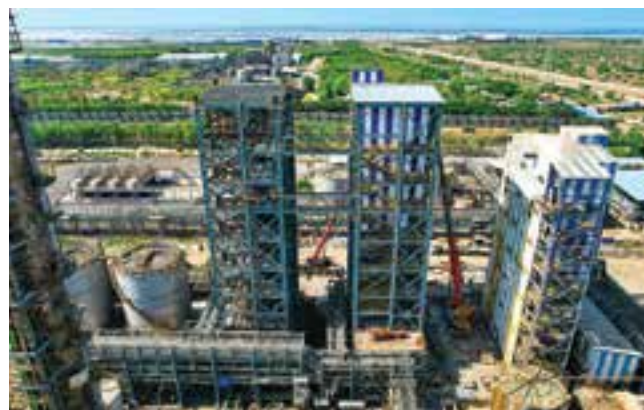
▲ Aerial view of the CNA 6 & 7 plant at Dahej.
