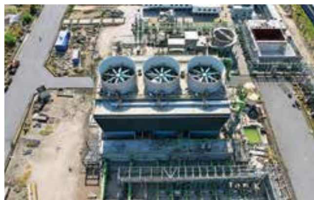
▲ Aerial view of the Cooling Tower at Dahej.
