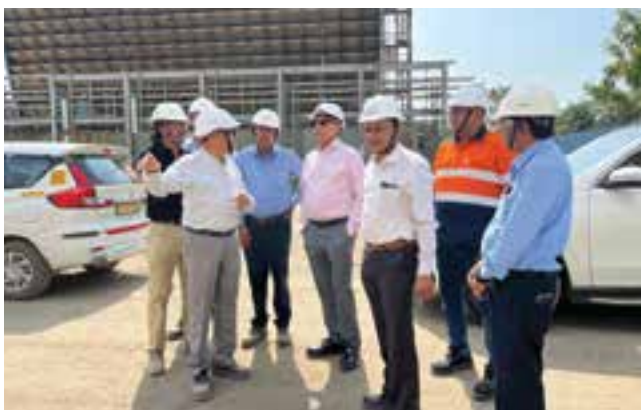
▲ Mr. S.C. Mehta, CMD – DFPCL, reviewing the progress at the Dahej project site.
