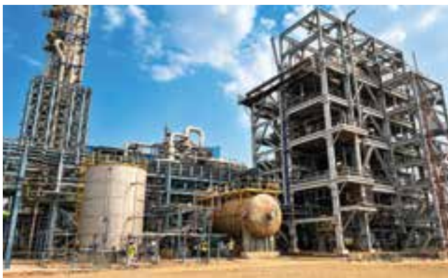
▲ Weak Nitric Acid plant nearing completion at Gopalpur.
