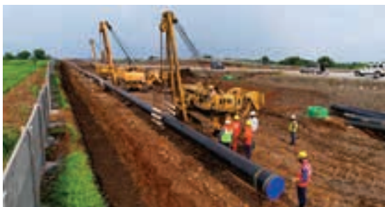
Laying of Natural Gas pipeline from Mumbai to Nagpur under MNGPL project
