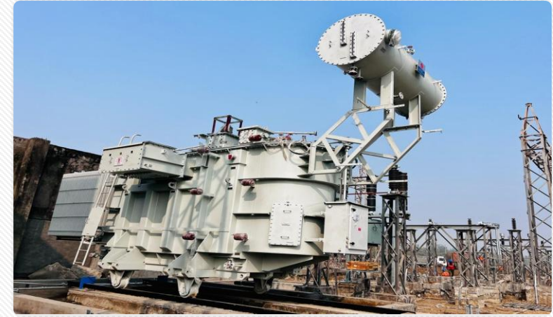
Power transformer installation completed
