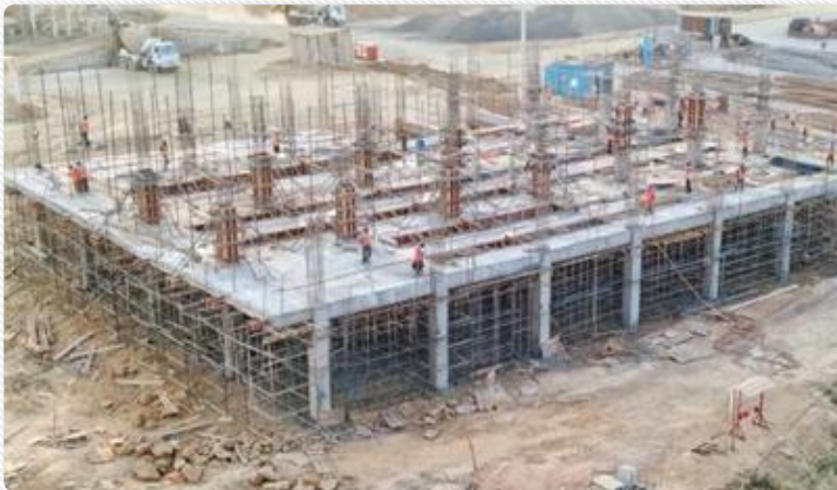
Load center 1 st slab casting completed
