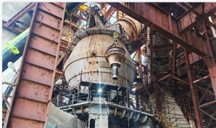
Raw Mill modernization work-in-progress
