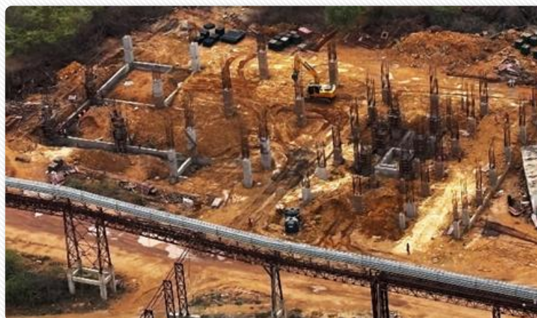
Kutch WHR – Turbine Generator and Air-Cooled Condenser building civil work-in-progress
