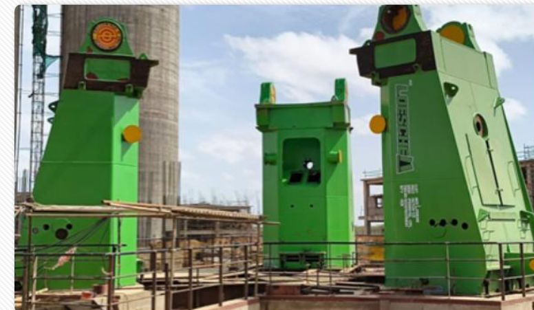
VRM installation commenced
