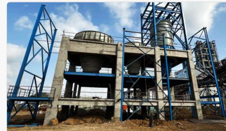
Hopper building structural work progressing
