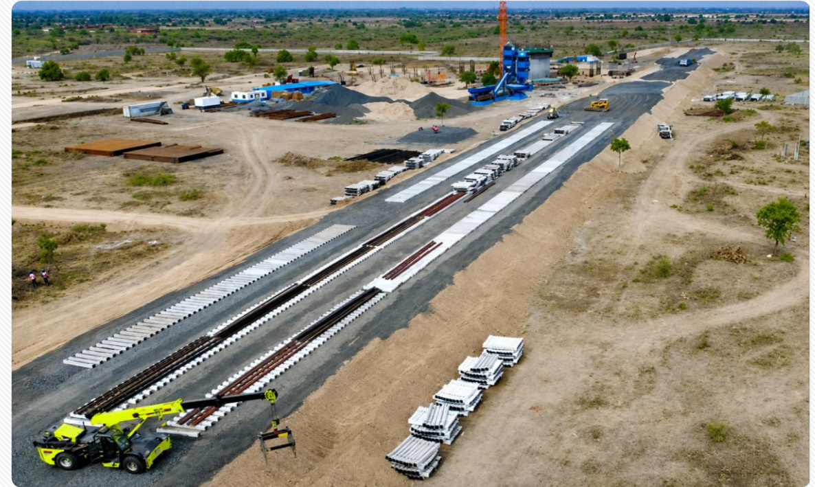
Railway Siding – Track Laying in Progress
