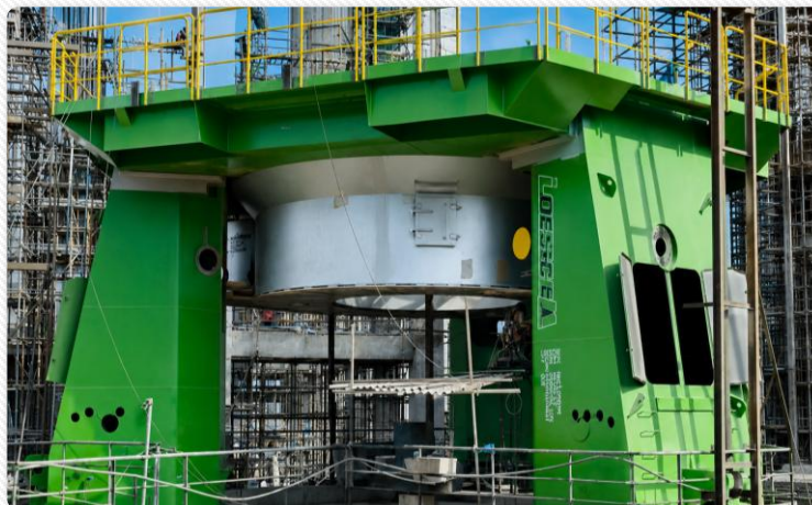
VRM Equipment Installation
