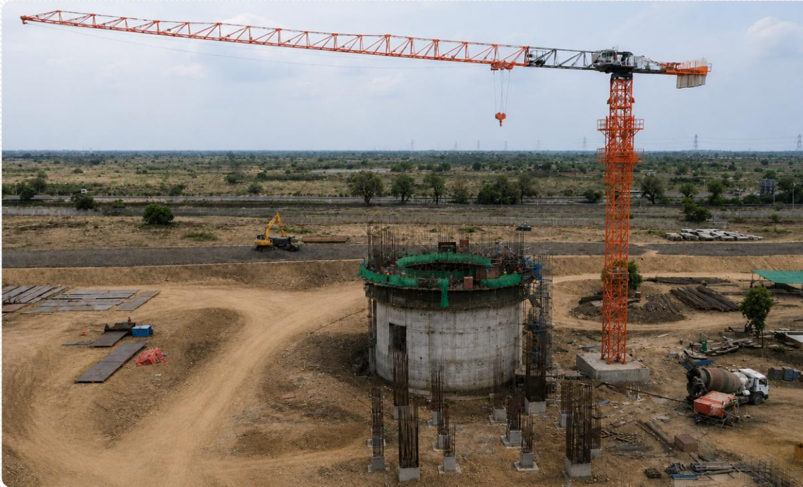
Silo Casting Work in Progress
