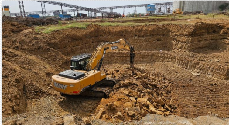
Kutch Grinding Unit foundation underway
