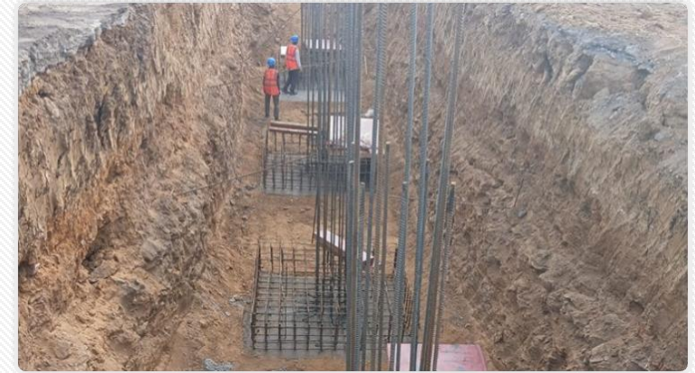
Hopper foundation work in progress at Kutch
