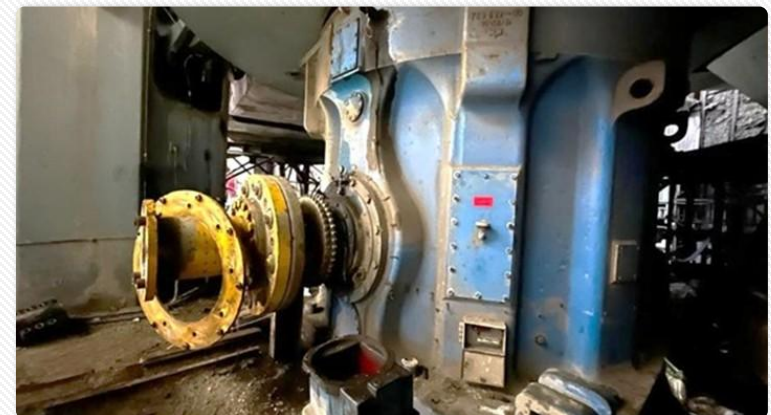
Raw Mill (VRM) HT Motor dismantling done at Surat
