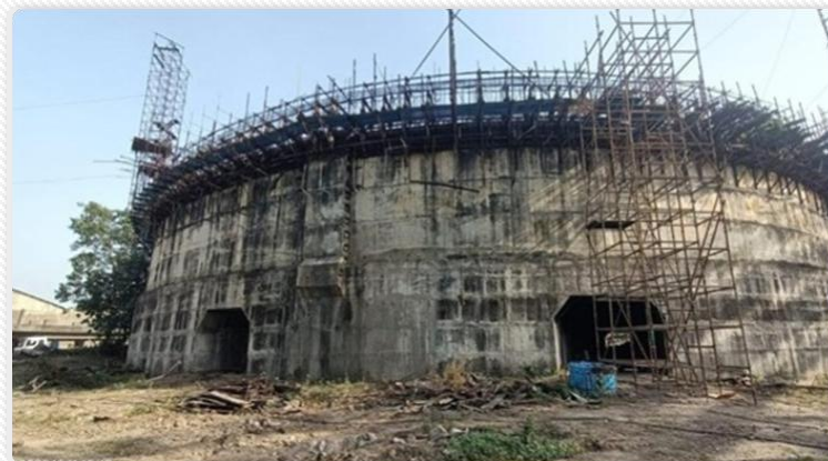
Fixing Slip Form for Silo construction at Surat
