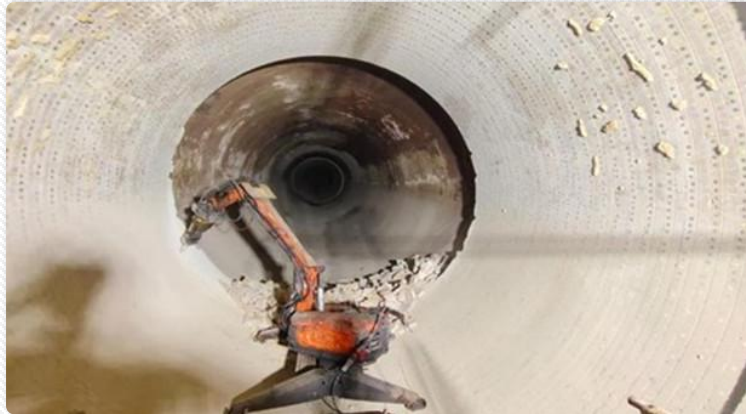
Kiln refractory de-bricking in progress at Kutch
