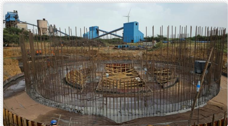
Silo base construction underway at Kutch
