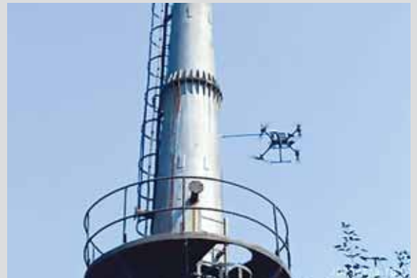
Using drones for smoke stack inspection at our industrial chimneys
