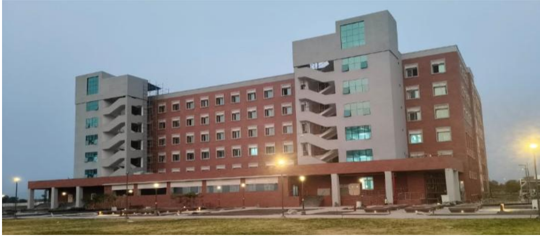
Construction of Shri Ramchandra Institute of Medical Sciences (SRIMS) College - Nursing College Building classroom in Aurangabad
