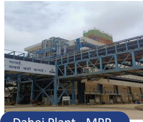
Dahej Plant - MPP
