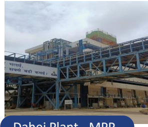
Dahej Plant - MPP
