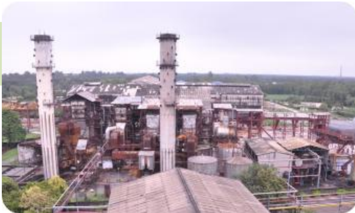
Sugar plant overview
