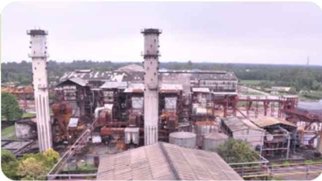
Sugar plant overview
