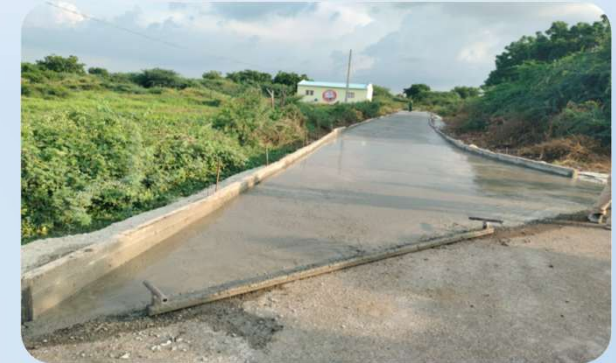
Laying of CC Road At Ramapuram Village, Dacheppalli, Andhra Pradesh
