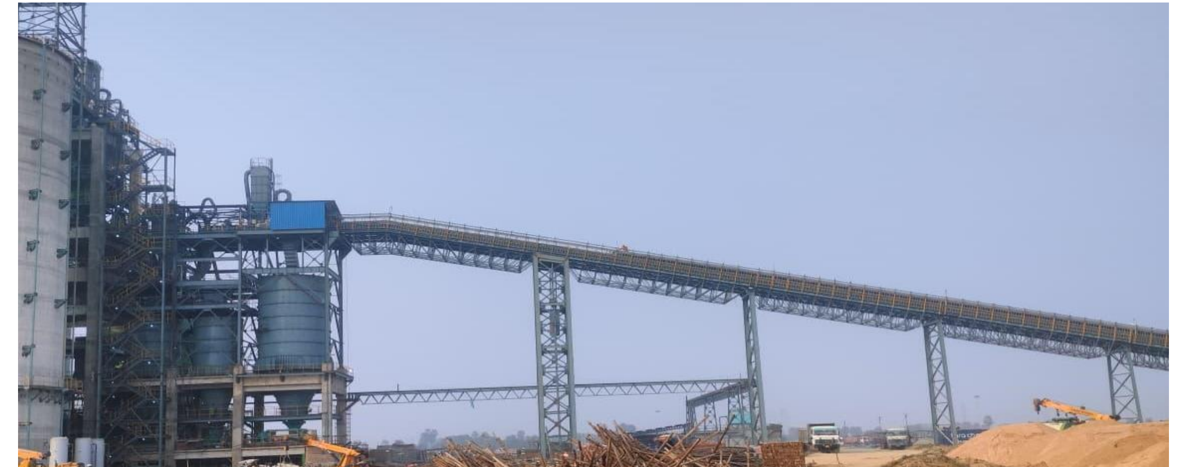
Hopper Building & Belt Conveyor
