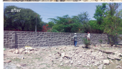
Repair of Boundary Wall
