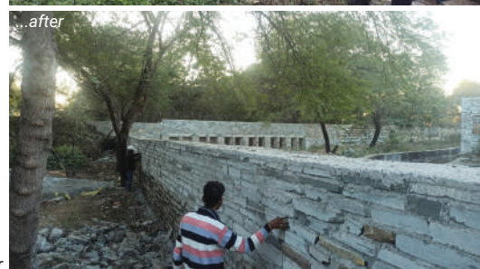
Construction of Boundary Wall and CC Work at Tejaji Mandir
