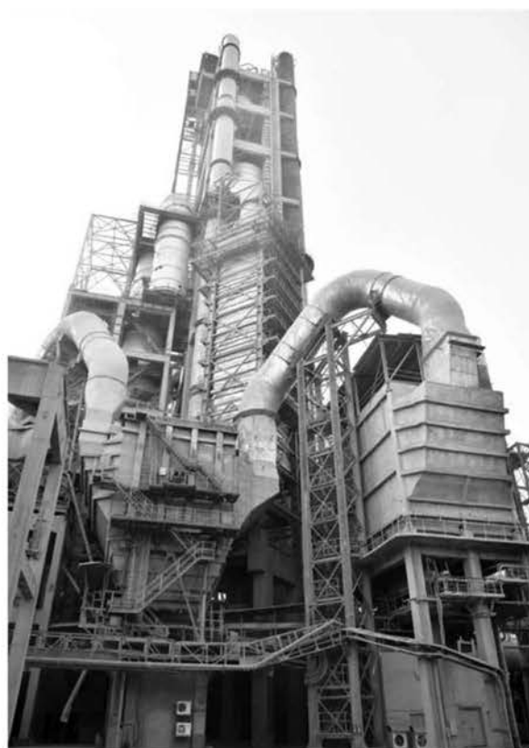
5 stage Pre Heater and Electrostatic Precipitator (ESP)
