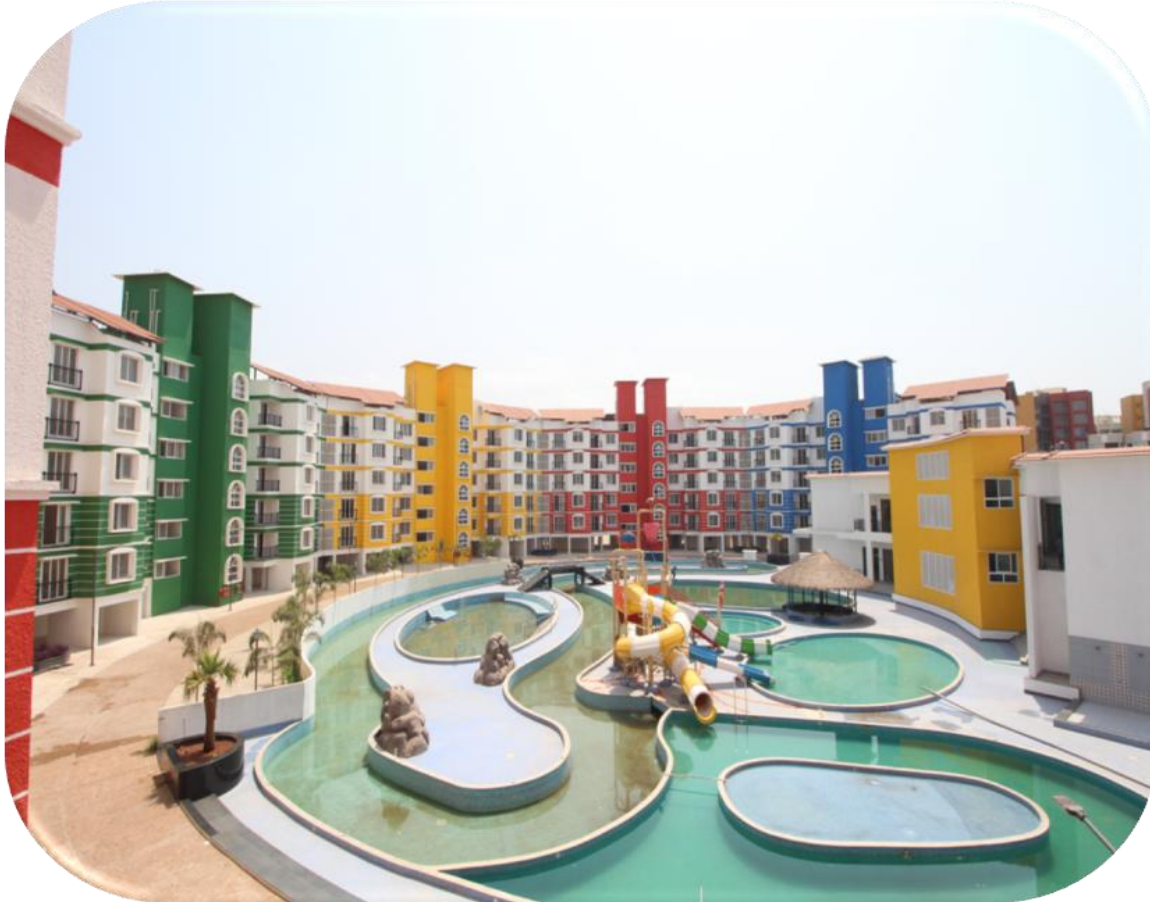
PROVIDENT ADORA DE GOA (received OC for Phase 1 to 6) Goa
