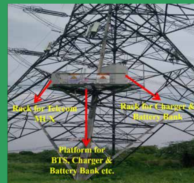
Technical Arrangement for Tapping of Induced Power in Earth Wire
