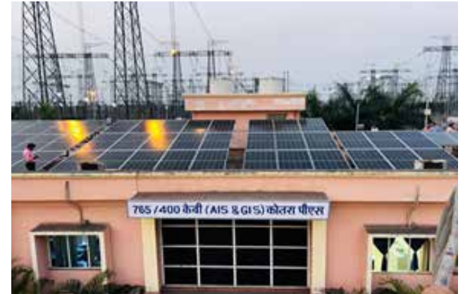
Roof Top Solar installation
