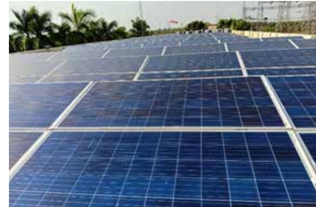
Roof Top Solar installation
