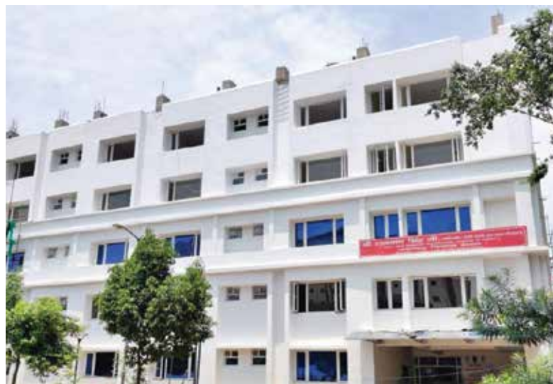
POWERGRID's Vishram Sadan, Lucknow
