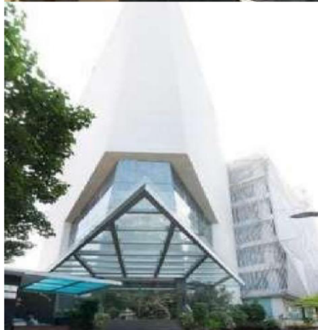
CCIL Bhavan Phase I Upto 6 th floor
