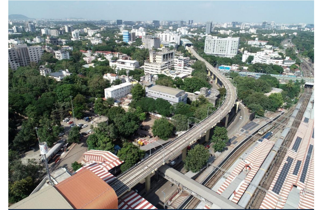
Pune Elevated Metro
