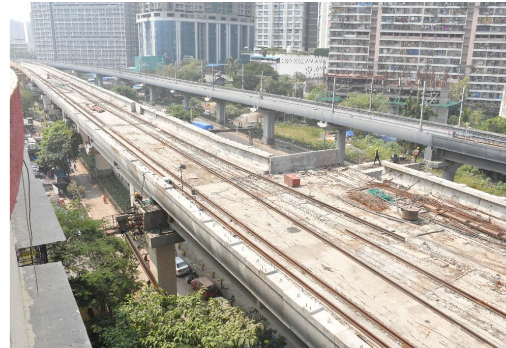
Mumbai Metro Line 9
