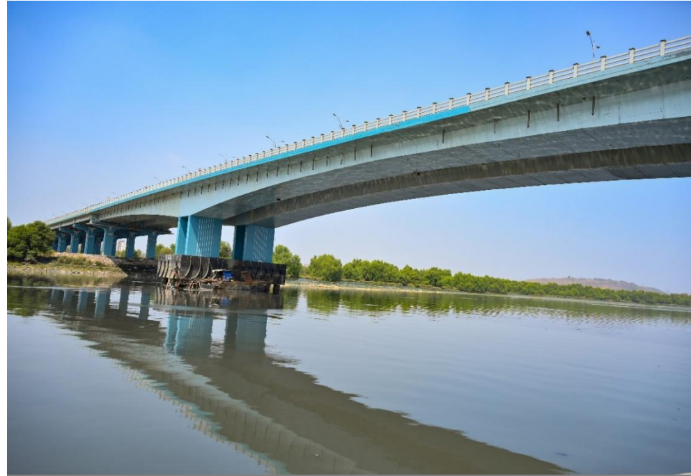
Motagaon Creek Bridge
