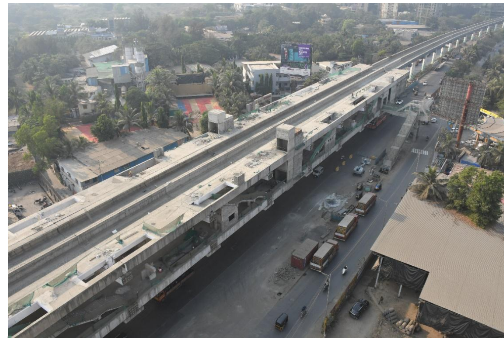
Mumbai Metro Line 4A
