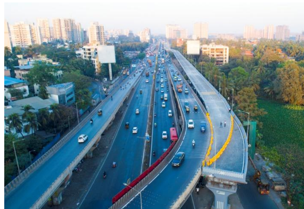
Chheda Nagar Flyover Part 1
