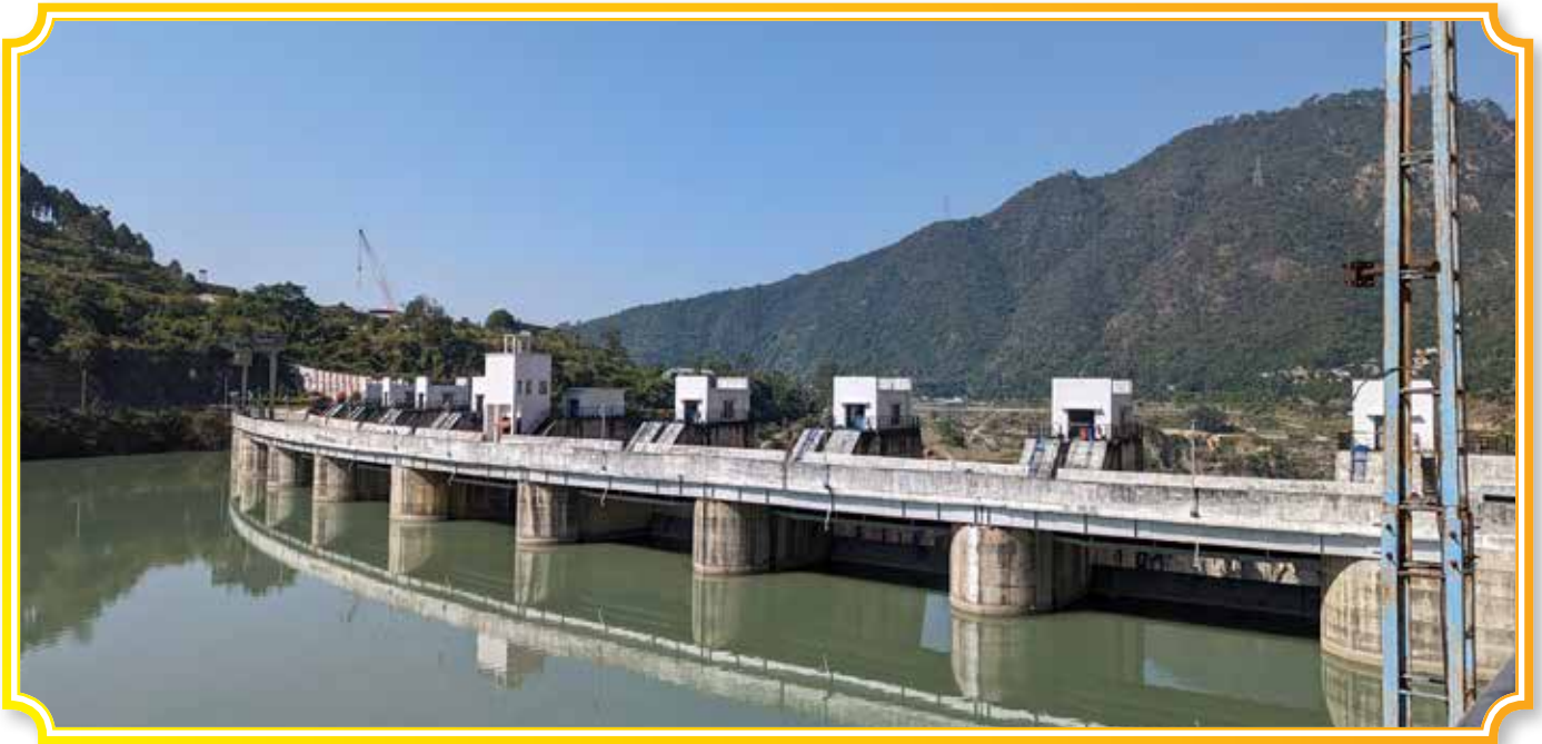
Dam & Reservoir of 4x82.5 MW Alaknanda Hydro Power Pvt. Ltd. (Uttarakhand) financed by REC
