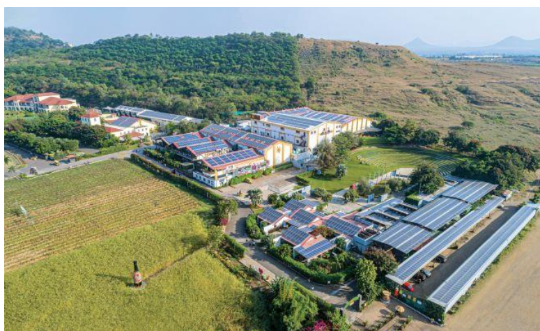
Our facility at Nashik, Maharashtra
