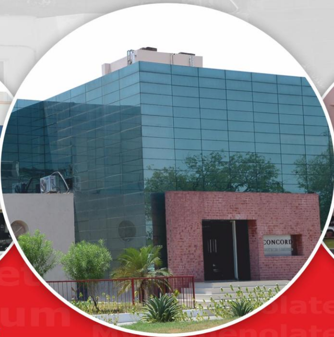
API Facility Dholka, Ahmedabad, India
