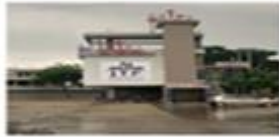
JTP-Hospitals- Muval – SCH (Secondary Care Hospital)
