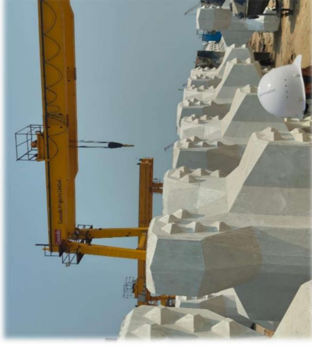
Works under progress at Jatadhhar site
