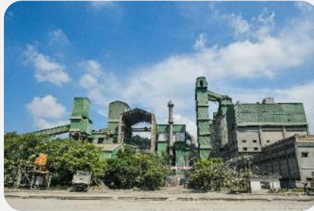
Guwahati Grinding Unit
