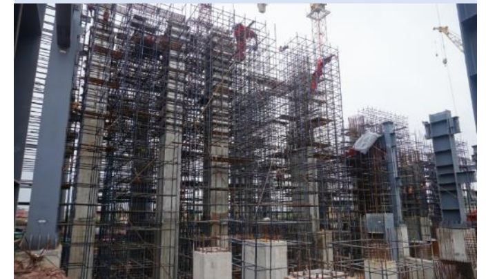
Unit #2 Turbine Generator Deck Column Casting
