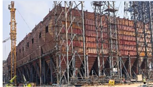
Induced Draft Cooling Tower
