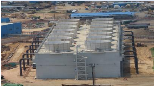
Induced Draft Cooling Tower
