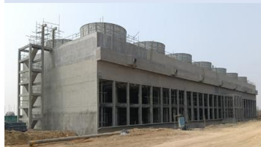
Induced Draft Cooling Tower
