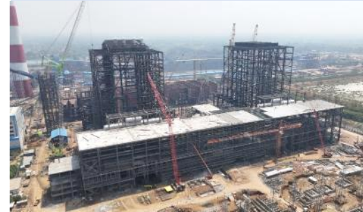
Unit #2 Electrostatic Precipitator
