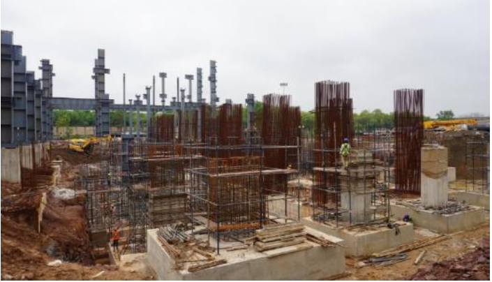
Unit #3 - Turbine Generator Deck
