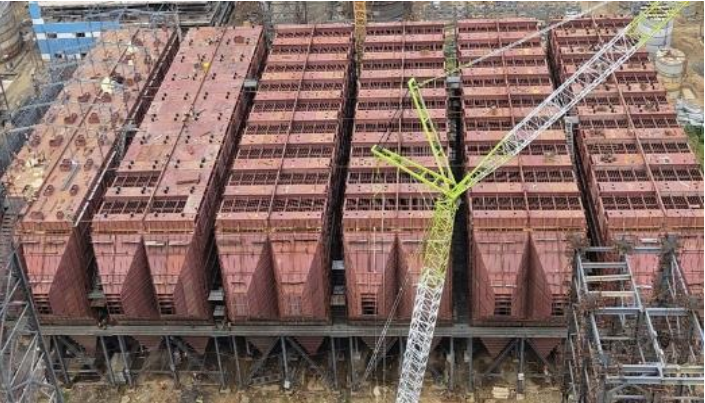
Unit #4 Electrostatic Precipitator
