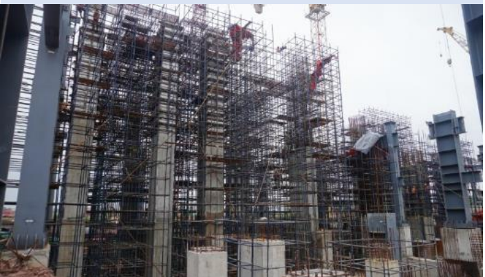
Unit #2 Turbine Generator Deck Column Casting
